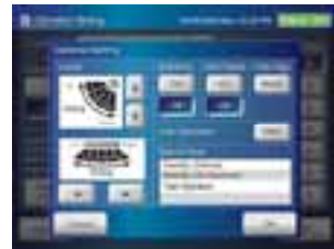
Indoor units operation monitoring
